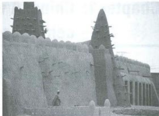
Source A: Mosque in Timbuktu, West Africa, completed in 1327. It is made almost entirely of earth and organic materials - fibre, straw and wood, and has prayer space for 2 000 people. It is still in use today.
